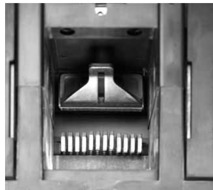
Magnum DS breaker contacts (arc chutes removed)
