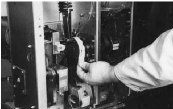
Figure 6-16 Remove Marked Masking Tape From Cam
