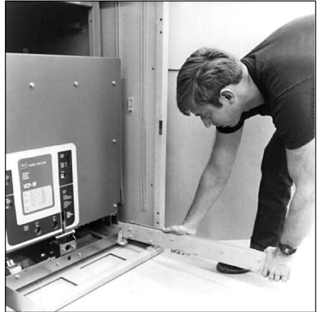
Figure 4-3 Engaging Extension Rails in a Lower Circuit Breaker Compartment
