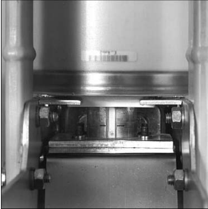
Figure 6-2 Vacuum Interrupter Showing Contact Erosion Indicator with Breaker Open (Shown Here for Clarity Purposes Only)
