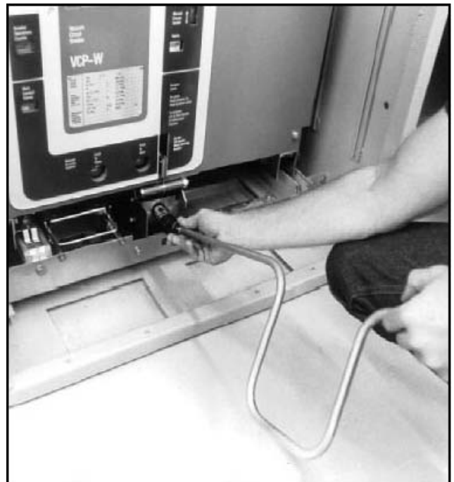
Figure 4-6 Engaging Levering-In Crank
