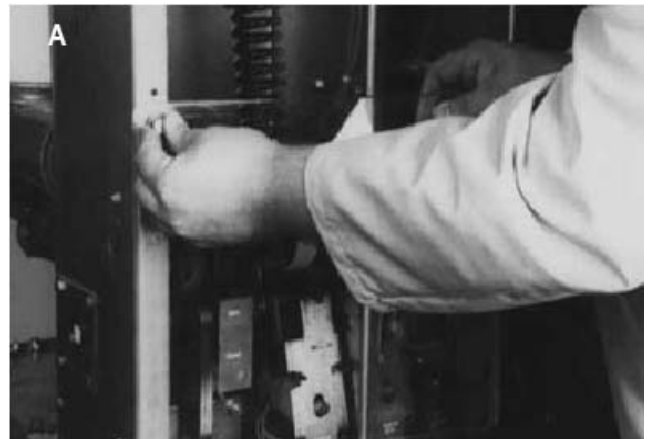
Figure 6-9 Attaching CloSure™ Test Tool at Hole “A”
